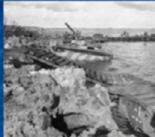
Seabees created the doodlebug to lay down ramps to help armored vehicles come ashore.
