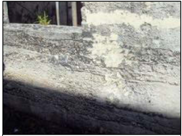
Layers of hand-mixed concrete comprise the bodega wall.
