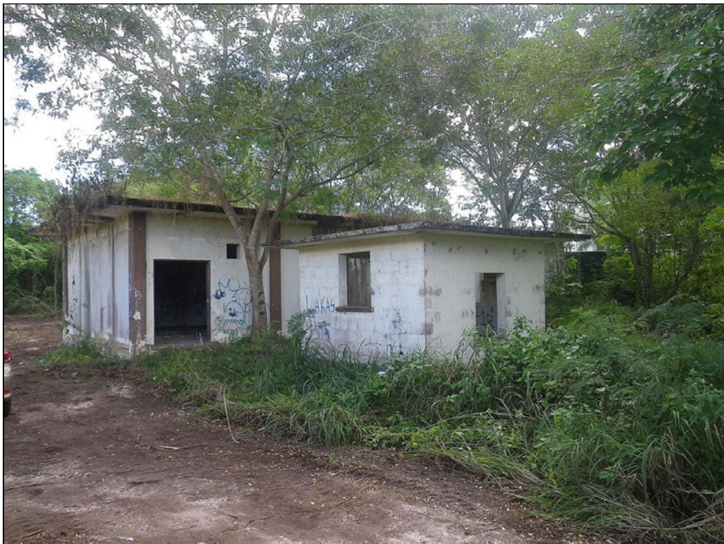
Figure 5. Generator Building. North and west side.
