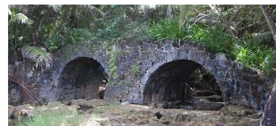
Left: Sella Bay Spanish Bridge (HPO 66-02-1002) was constructed in the late 1700s. The bridge measures 94 ft long by 9 ft wide. It is a double-arch structure over the Sella River and is located in a forested area just inland from the beach. The bridge is in fairly good condition.
