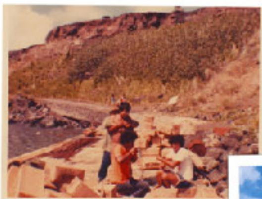
Unloading Cargo at Pagan dock
