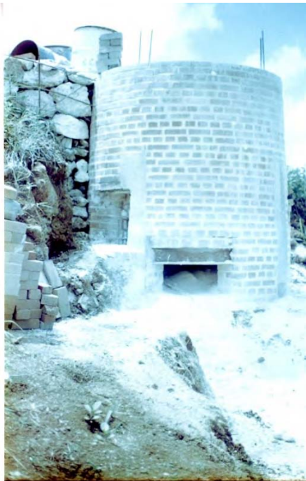
Figure 18. This photograph shows the kiln constructed to manufacture the mortar and stucco for the Soledad restoration.
