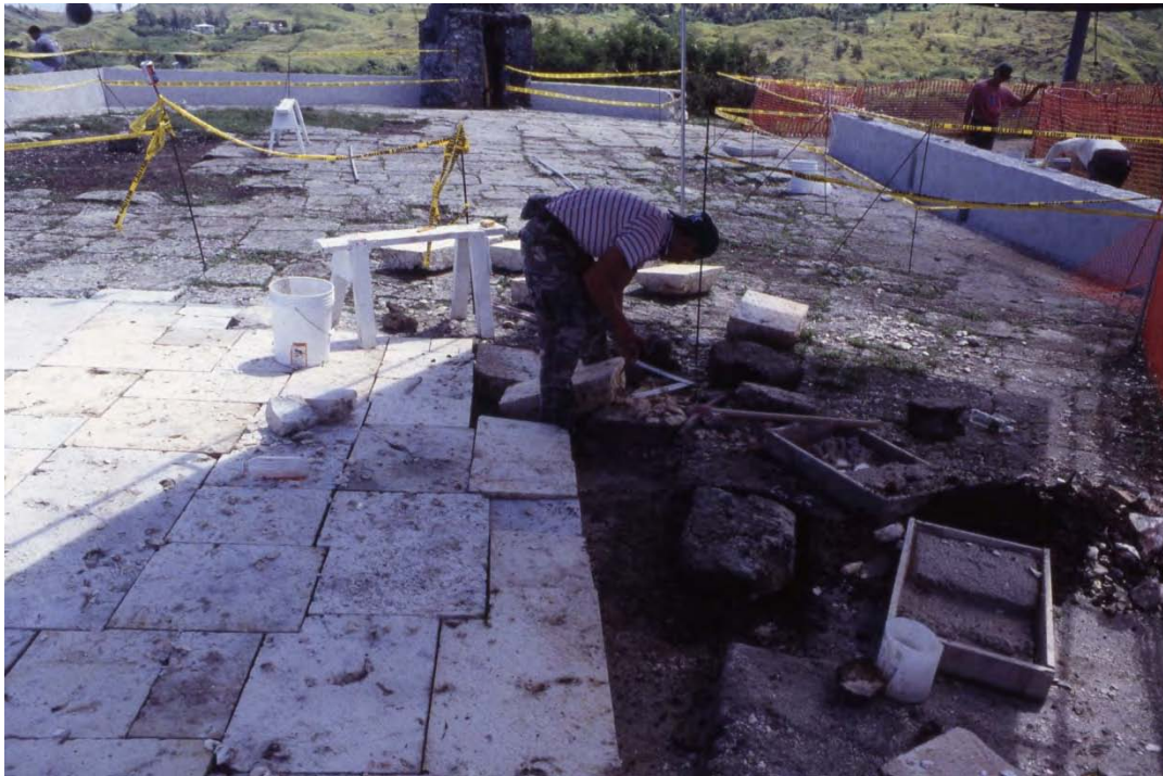
Figure 20. Photograph of one of the canteros fitting stones into the terraplene. Not only did the masons have to dress the stones, but they also had to prepare the base course. Note the mix of stone sizes and the intricate joinery, both in keeping with the original workmanship.
