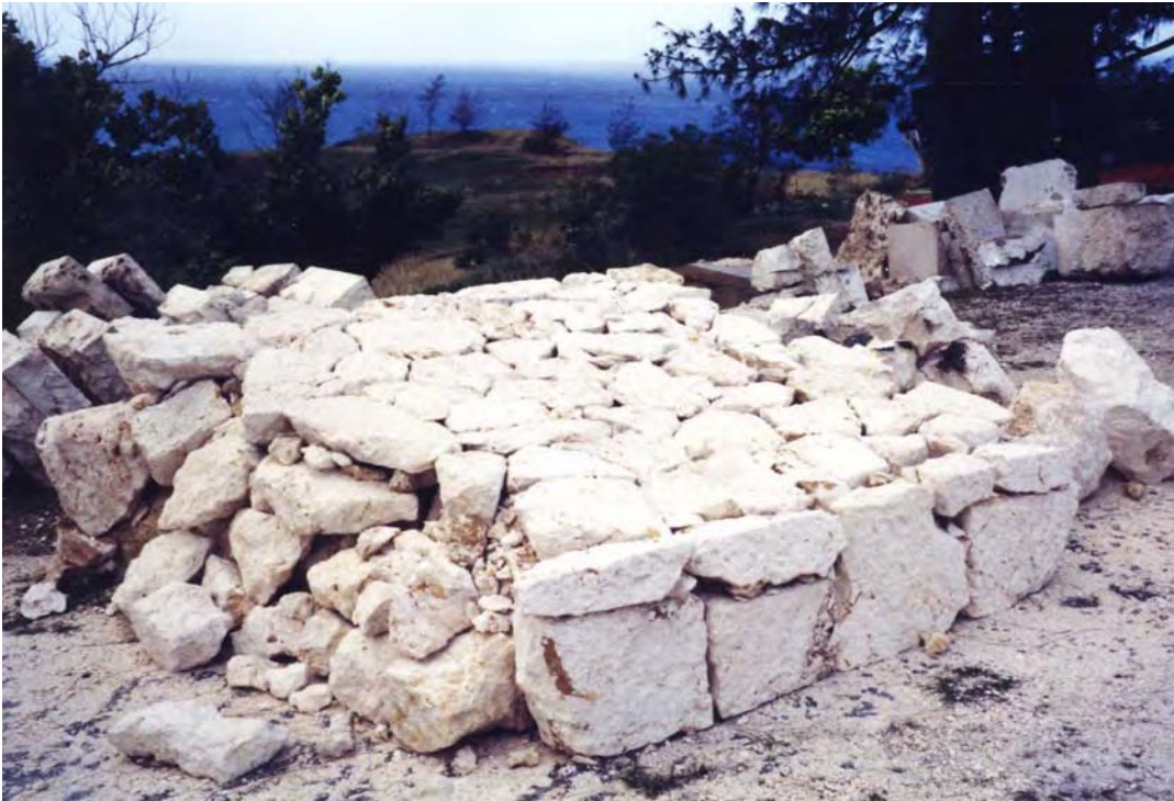
Figure 21. Photograph of one of the mock-ups of the finished barbette wall. This was built at a 1 to 1 scale.
