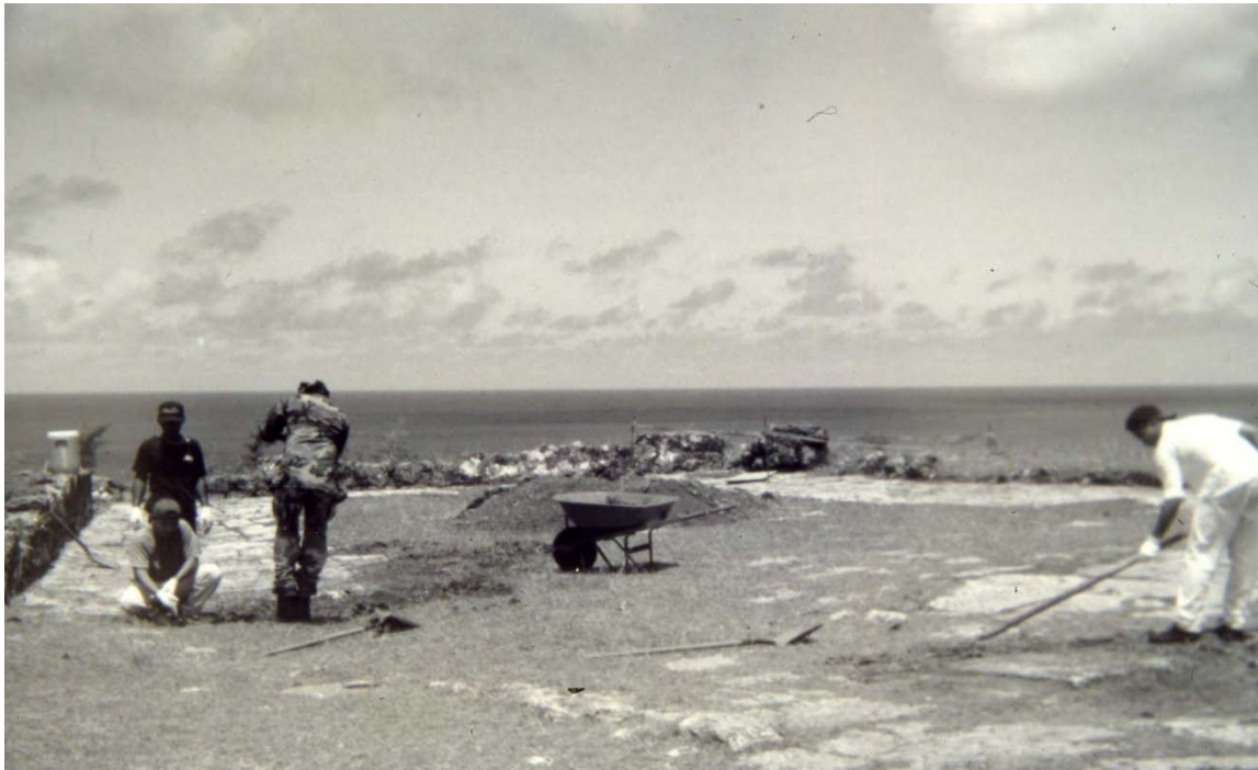
Figure 13. View to the south showing the crew removing soil and grass from the terraplene. The man on the right is using a fusiño .
