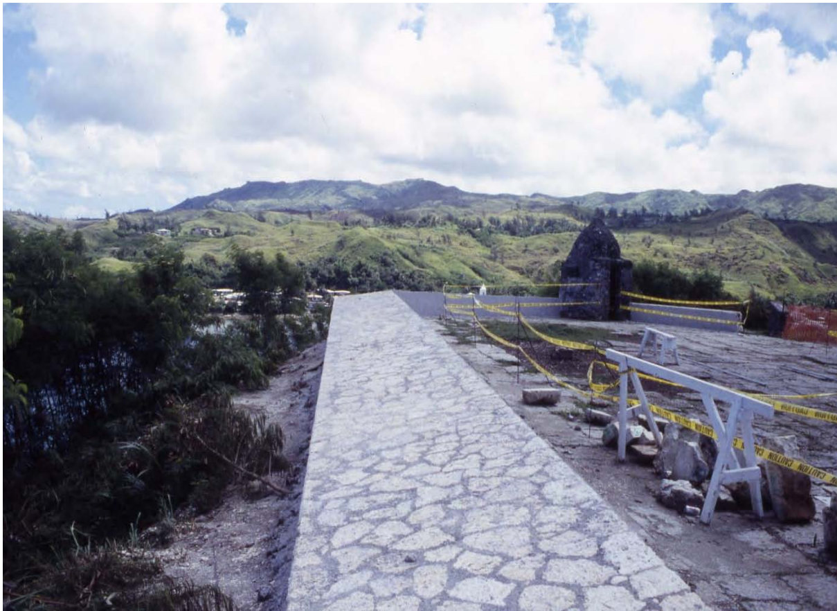
Figure 23. Photograph of the completed, west barbette wall prior to being stuccoed. Work on the garita has yet to start. This is the same stretch of wall that is pictured in Figures 12, and 22.
