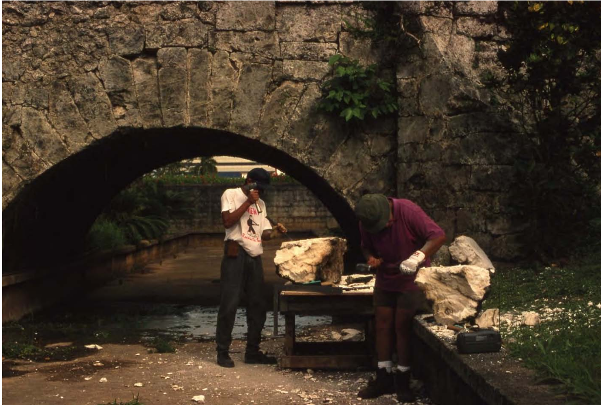
Figure 16. Photograph of Nicanor and Jose Luis Nequis in Hagåtña, dressing stone to repair one of the San Antonio Bridge buttresses. The characteristic tools of the mason, a level table, mallet, chisel, and square can be observed in this photograph.
