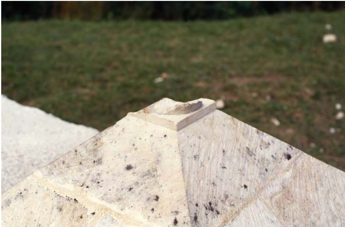
Figure 26. Close-up photograph of the broken ball finial on the gate pier cap.
