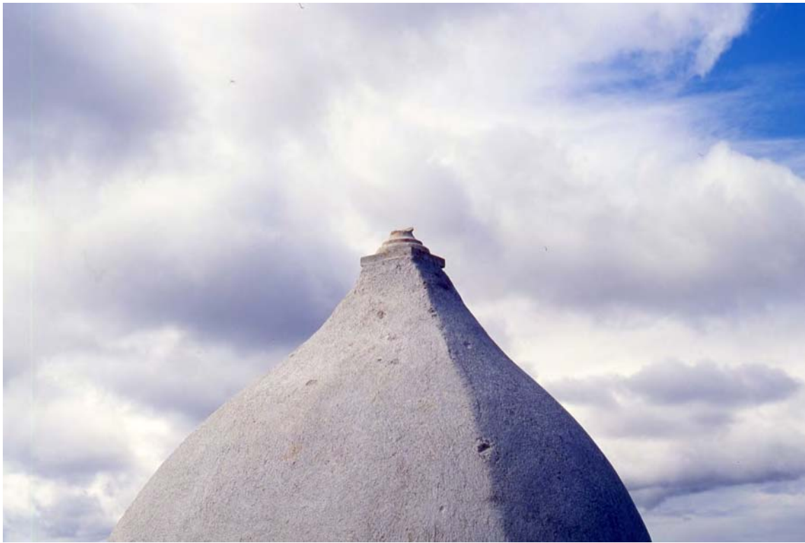
Figure 27. Photograph of the broken ball finial on the top of the garita.
