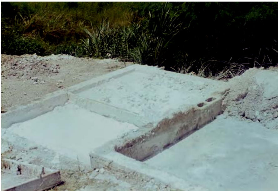
Figure 19. This is a photograph of the testing area that was used for the lime that was manufactured on site. Different qualities were needed for the stucco than were required for the mortar to be used in mamposteria construction.
