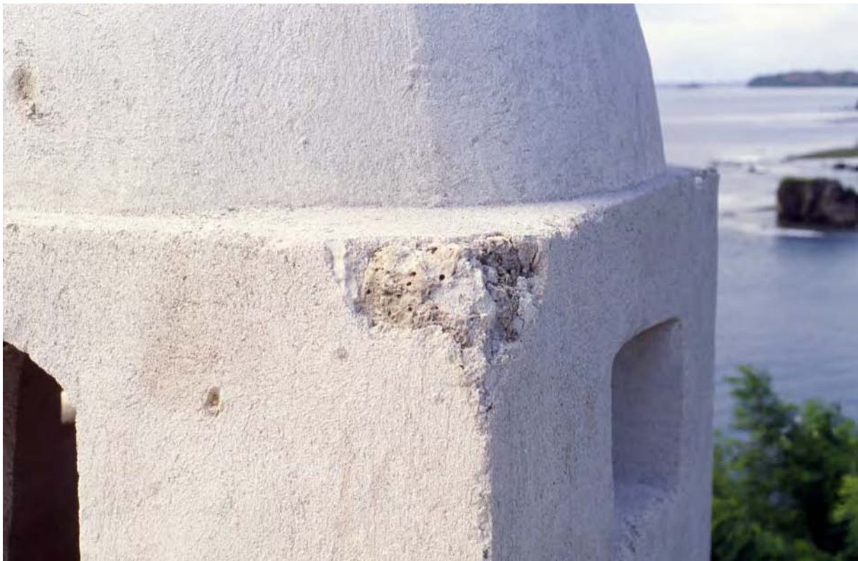
Figure 28. Photograph of damage to the southeast corner of the garita.
