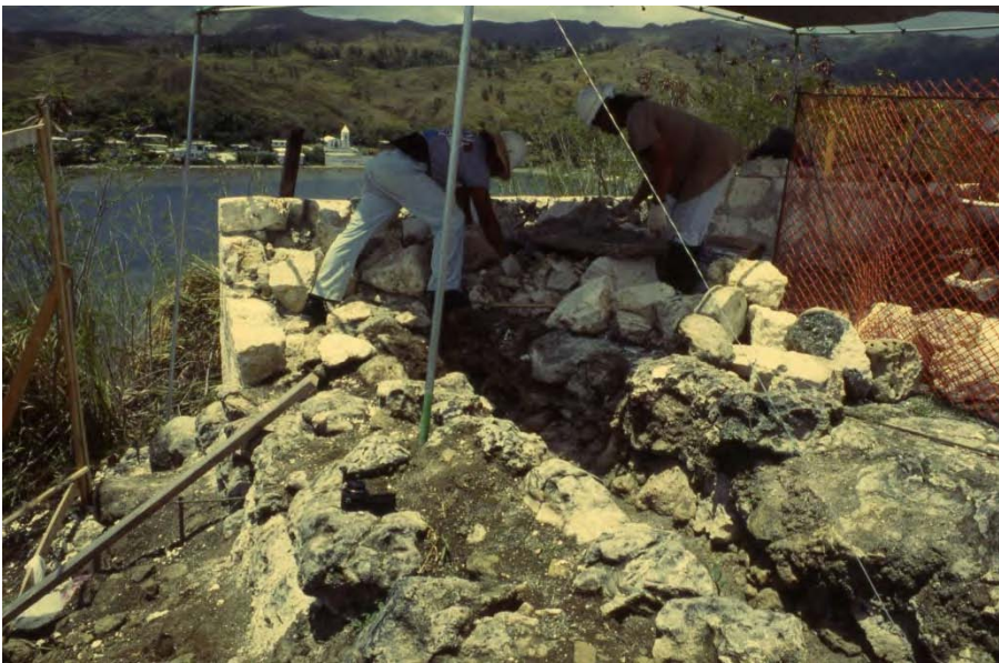
Figure 22. Photograph of work on the northwest barbette corner.
