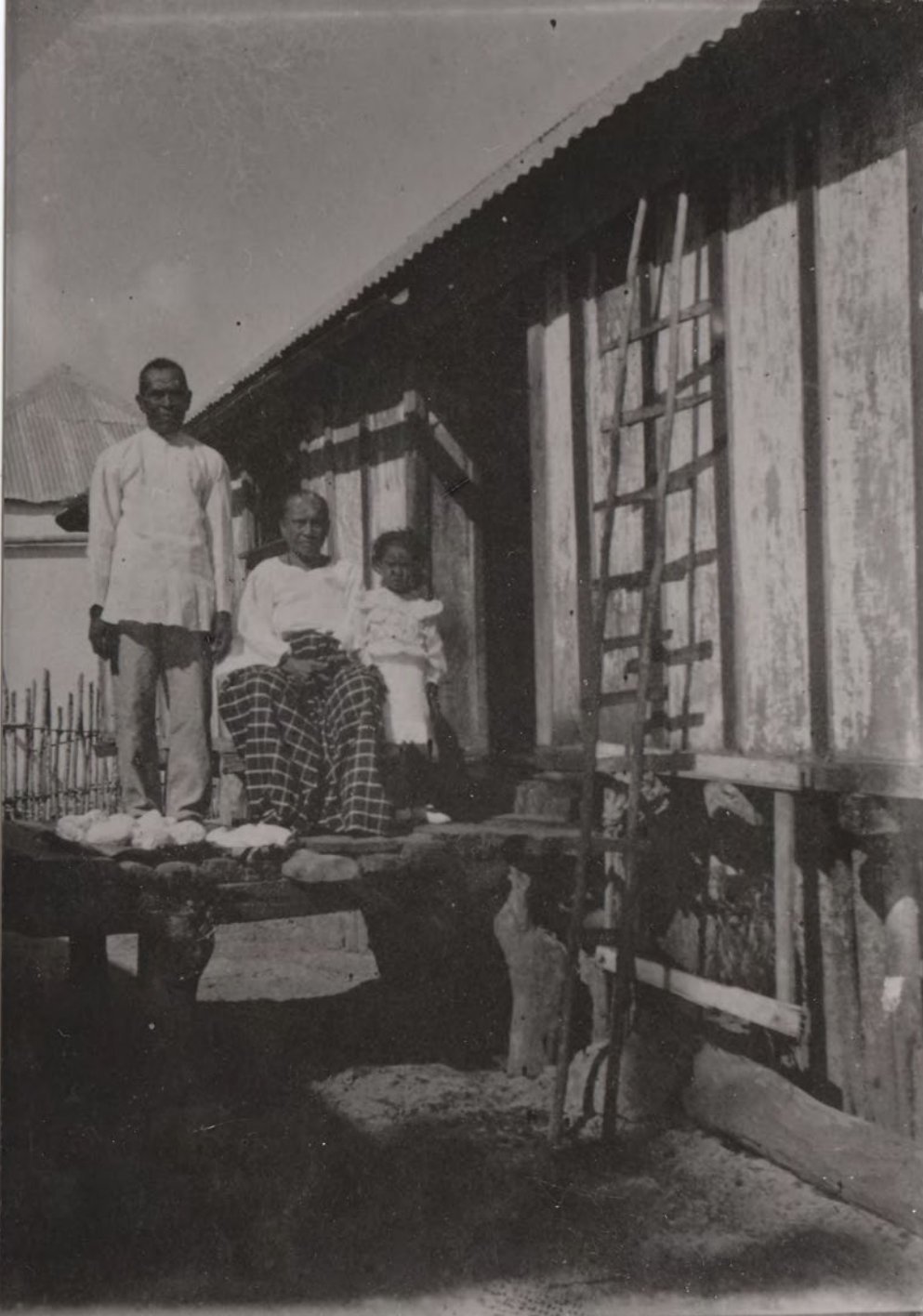
A wooden batalan linking a Chamorro residence with the kitchen. Similar batalan were used in mampostería architecture (Fritz Collection).
