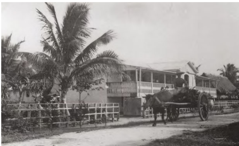
The Ada residence, circa 1905 (Fritz Collection).
