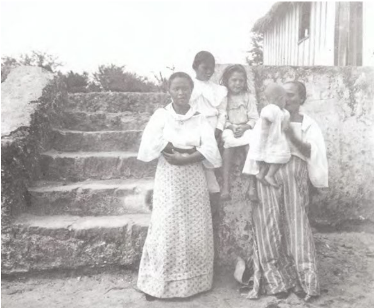
A massive stone stairway typical of mampostería architecture (Fritz Collection).
