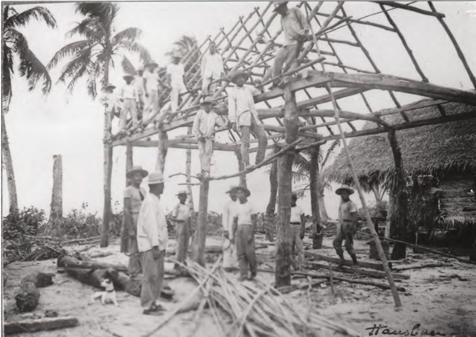
Workers erect the wooden frame of a traditional Chamorro residence (Fritz Collection).
