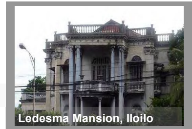
Figure 1: Spanish Colonial Structures Made of Coralline Limestone
